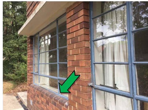
Photo 4. Exterior, southern elevation, window frames – assumed non asbestos containing window caulking.
