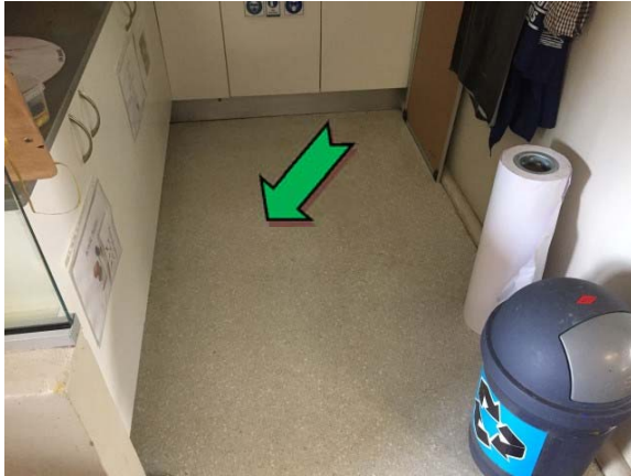
Photo 7. Interior, laundry, white floor coverings – non asbestos-containing vinyl sheeting.
